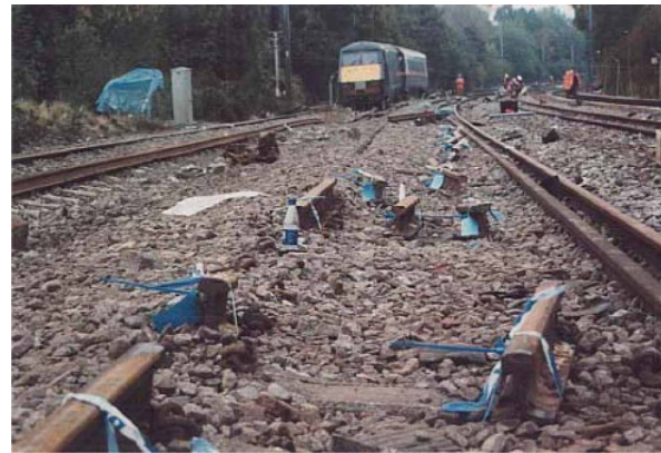
Fig. 6 The Hatfield rail track site (taken from reference [31])
